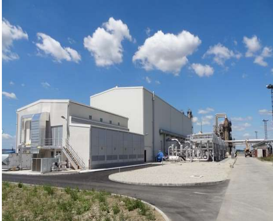
Figure 3. CO 2 Compressor station on GPF Molve
