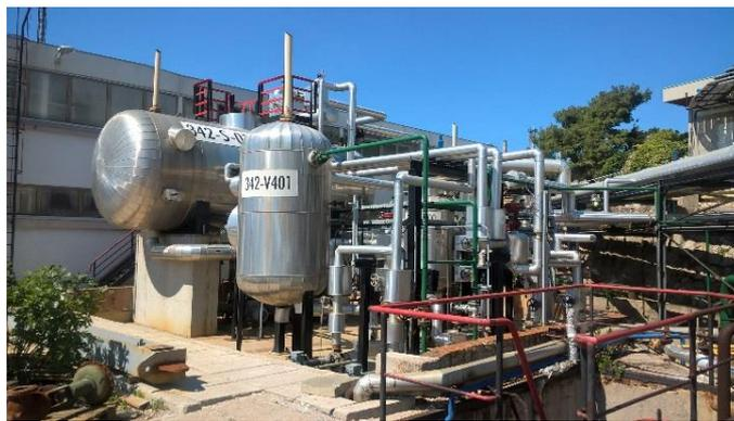
Fig. 3 Central condensate collecting station with heat exchanger and condensate tank
